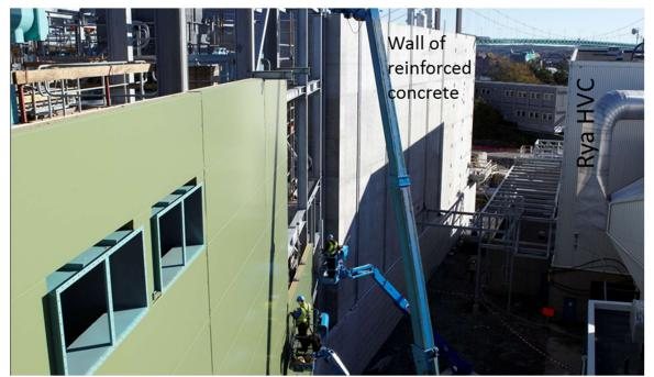
Figure 2.3: Illustrating the proximity to the neighboring plant Rya HVC and the constructed wall of reinforced concrete.
